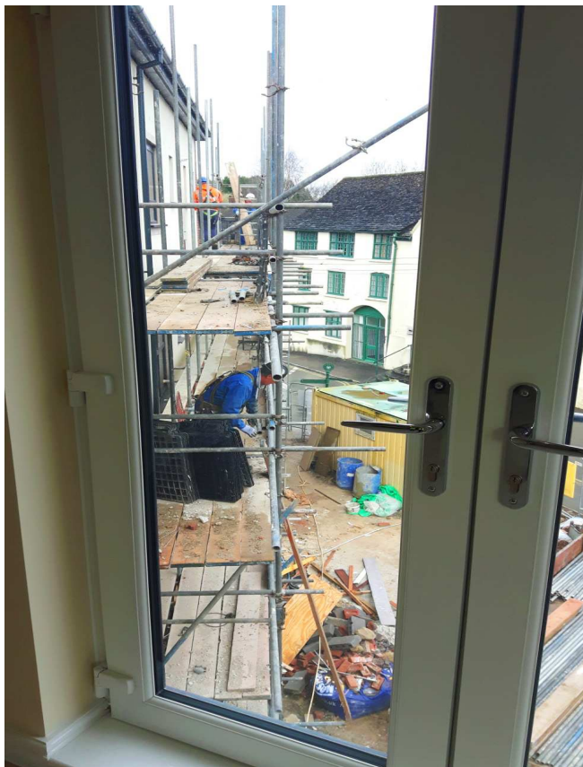
Affordable flats under construction at Dursley, 2017
