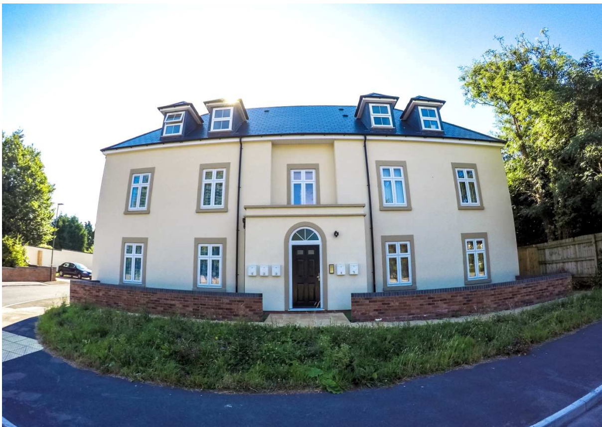
Affordable flats in converted former hotel, Newport, Berkeley.
